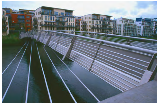
Figure 12.12. The Apaté bridge in Stockholm uses duplex 2205
