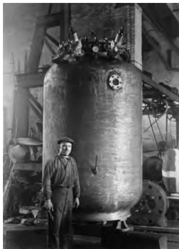
Figure 12.2. Autoclave in 453S for the production of gunpowder, delivered in 1933
