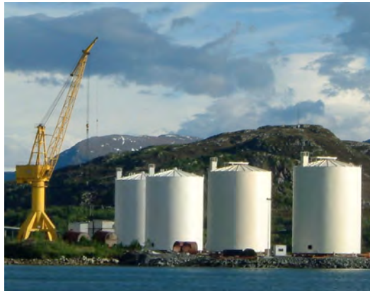
Figure 12.10. Storage tanks built in LDX 2101®
