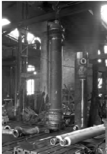
Figure 12.1. Brobeck cooler, fabricated in 453S for a sulfite mill, delivered in 1932
